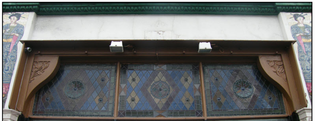
The decorative coloured glass between the two sets of decorative tiles above the doorways as seen from outside the building. One can only imagine how attractive this must when seen from inside the building!
