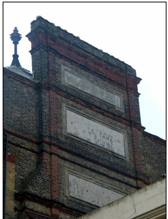
The massive chimney stack to the north side with fifteen chimney pots. The purpose of the metal erection on top of the building is unknown but it has been suggested that it might have been placed there to mark a higher point than the top of St John's Church steeple that was built at around the same time as the Man of Kent
