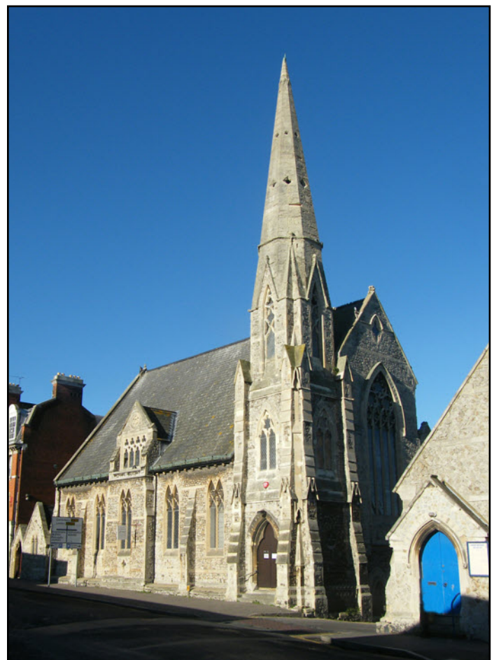
The former Congregational Church in Union Crescent . The church was built in 1860. A corner of the former Sunday school building can be seen on the right of the picture
