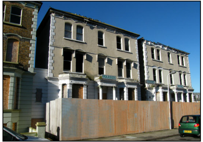
The fire-damaged structure of the Warren Court Hotel. The controversial proposed redevelopment of the south side of Dalby Square would see a reinstatement of a terrace and the retention of the façade of the Warren Court Hotel
